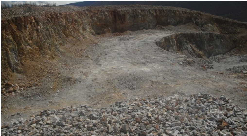
Figure 63 Commencement of the construction of a bench
