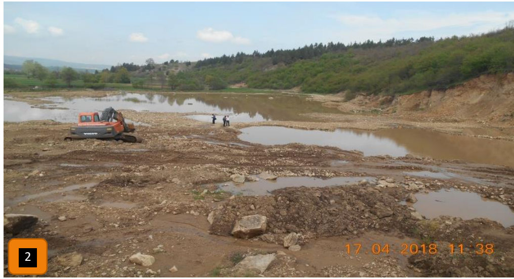
Figure 22 Mining of inerts in the river, damage to the floor layer of Mirusha riverbed - ICMM
