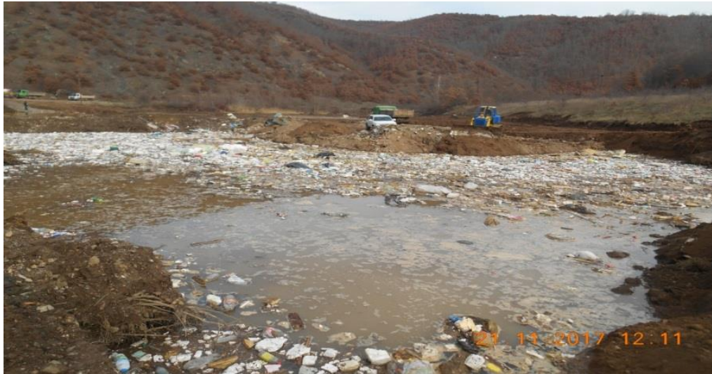
Figure 68 Recultivation-filling with waste of mined holes - contamination of land with urban waste – Municipal inspectorate
